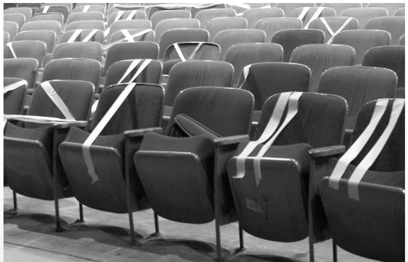
Many of the seats in the High School auditorium are broken, limiting the availability of seating for High School musicals, band performances, and district-wide school concerts. Auditorium restorations are part of the proposed capital projects referendum.
